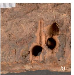
Fig. 2 e-h e, f and b) Small wooden wedges with animal glue and filling mass; g) texile (flax) as filling material; h) cubically shaped holes for dowels 8-10 mm.
