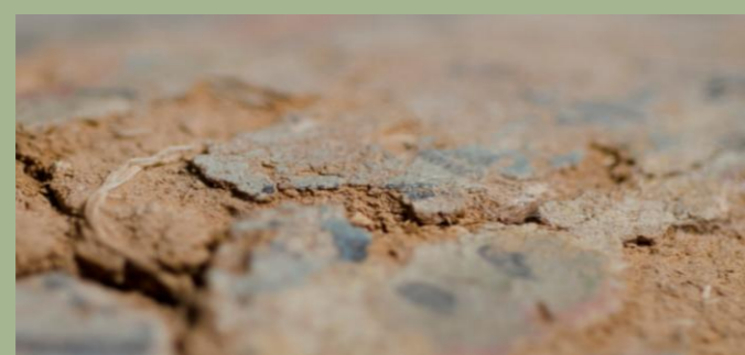
Fig. 10: Detail of the painted stola. Note the fiber integrated in the adobe at left.
