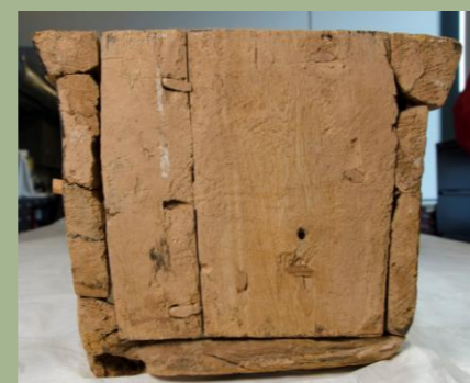
Fig. 4: Nine wood elements converge at the unpainted base.
